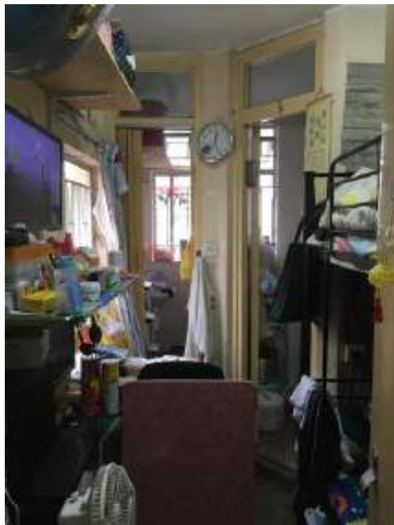
改造前 Before renovation
