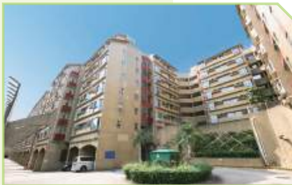
▲ Trackside Villas 策誠軒
