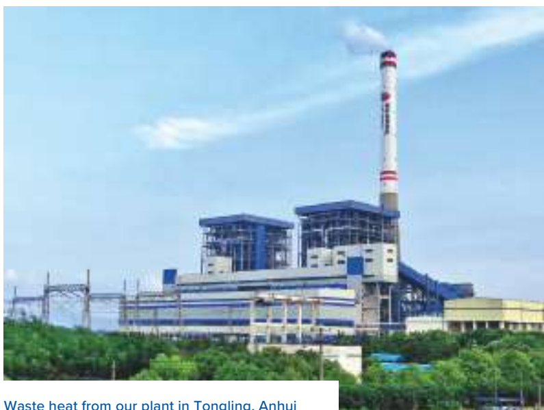
Waste heat from our plant in Tongling, Anhui province is converted into energy for use by our industrial customers.
