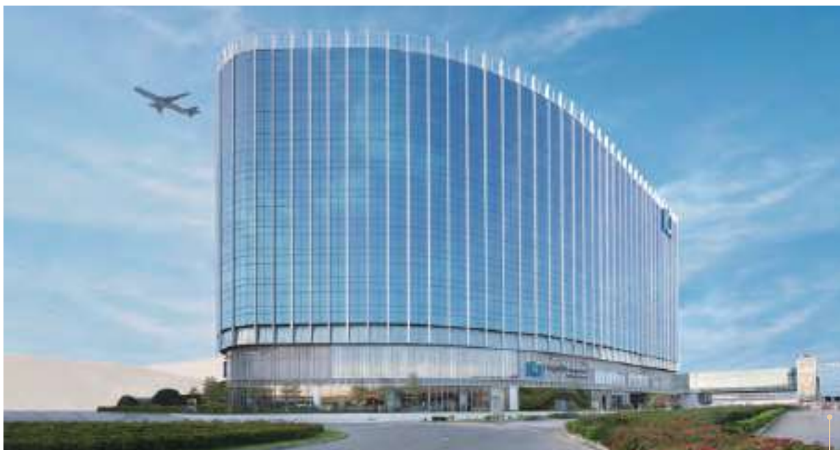
Town gas hot water boilers provide stable hot water supply for the brand-new Regala Skycity Hotel.
