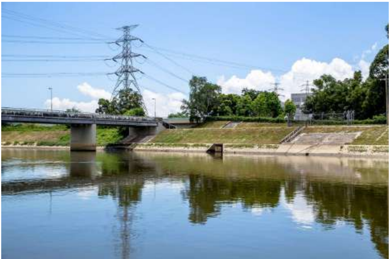
Maintaining proper Health, Safety and Environment management practices for transmission towers is important to keep the general public safe.
