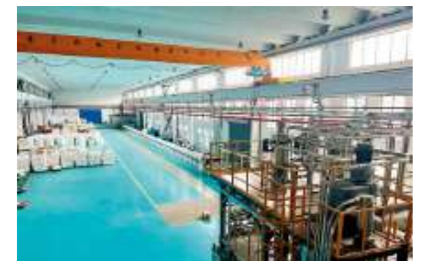
CR Chemical Materials' PET foam production line
