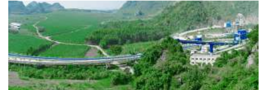
Green Mine Construction of CR Cement Pingnan Company
