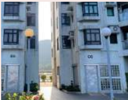
Floodgates were installed entrances and plant rooms in building blocks that are located near the coast and basement carpark
