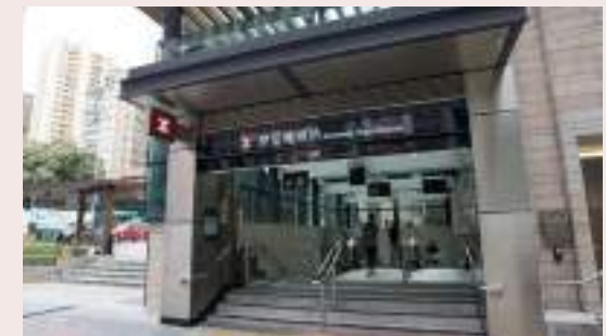
The entrances/exits of most MTR stations are by design at least 450mm above street level and equipped with 1.2m high flood boards.
