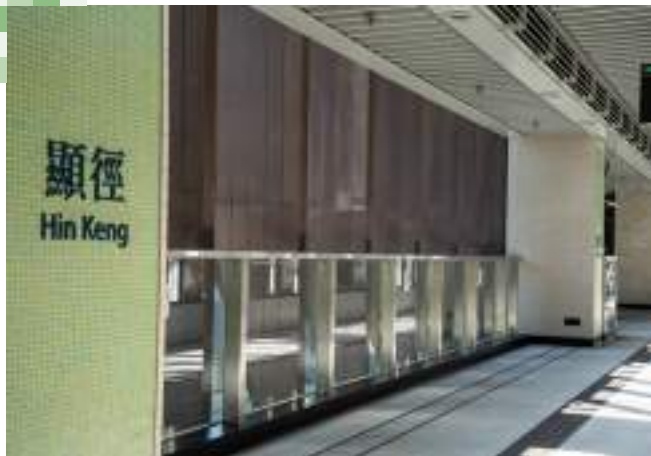
Solar shading devices made from environmentally friendly materials to shield passengers from sunlight, and the extensive green roof to reduce the indoor temperature at Hin Keng Station.
