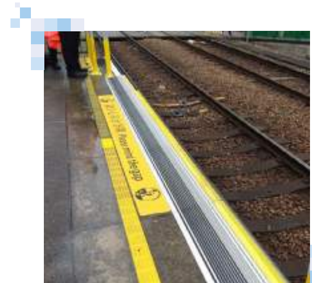
We install Board-Easy Mats or a ramp at Light Rail platforms with a large vertical gap to enable wheelchair users or people in need to easily board and alight our LRVs.
