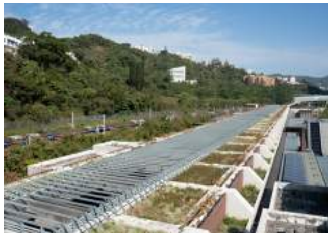
Solar shading devices made from environmentally friendly materials to shield passengers from sunlight, and the extensive green roof to reduce the indoor temperature at Hin Keng Station.
