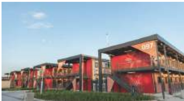
Temporary quarantine facilities at Penny's Bay
