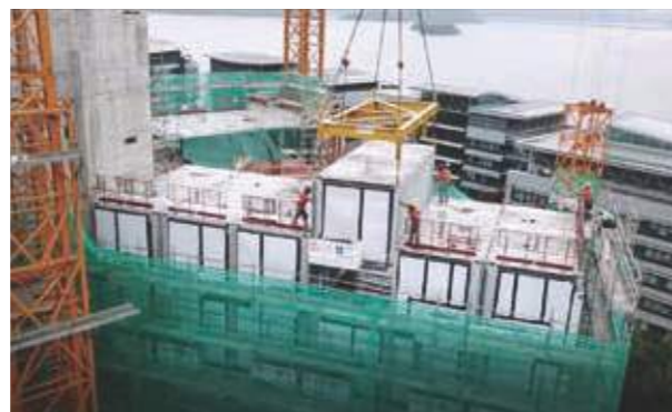
On-site installation of modules manufactured in factories
