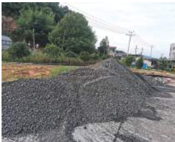
Collected waste bituminous for recycling
