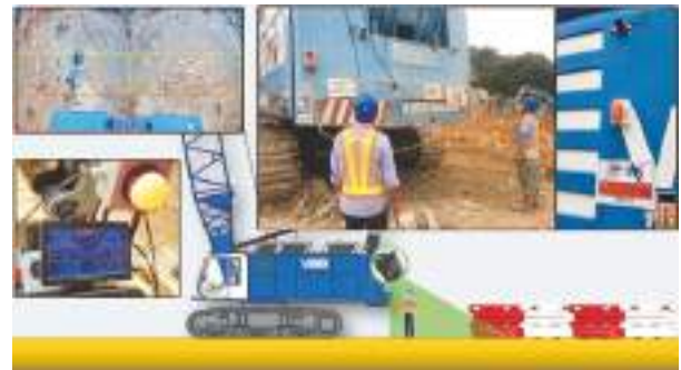
Danger zone alert system adopted to enhance site safety
