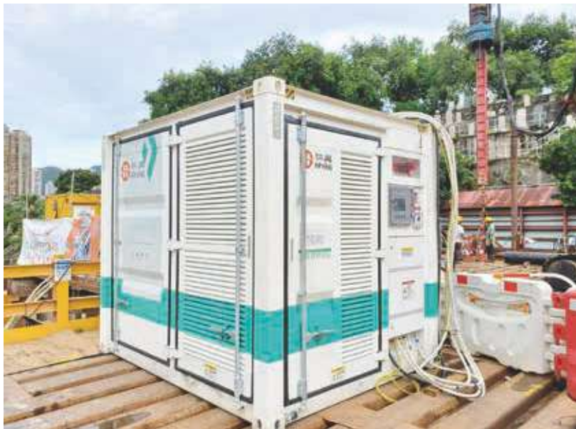
The BESS replaces the conventional diesel generators
