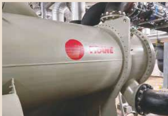
Two 2500TR chillers replaced in FY2022
