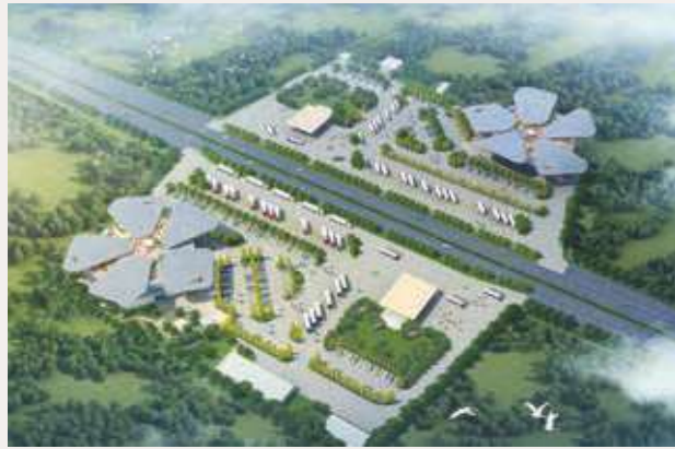
Use of UAV for road inspection
