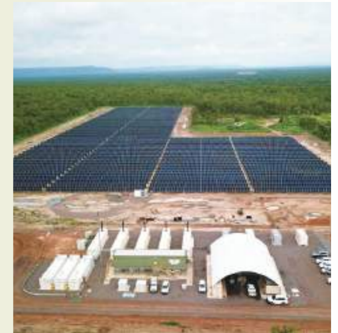
∞ Jabiru Hybrid Renewable Energy Project's battery and diesel power station
