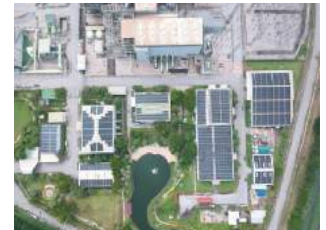
Ratchaburi Power’s rooftop solar system supplies electricity to the facility’s auxiliary power system.
