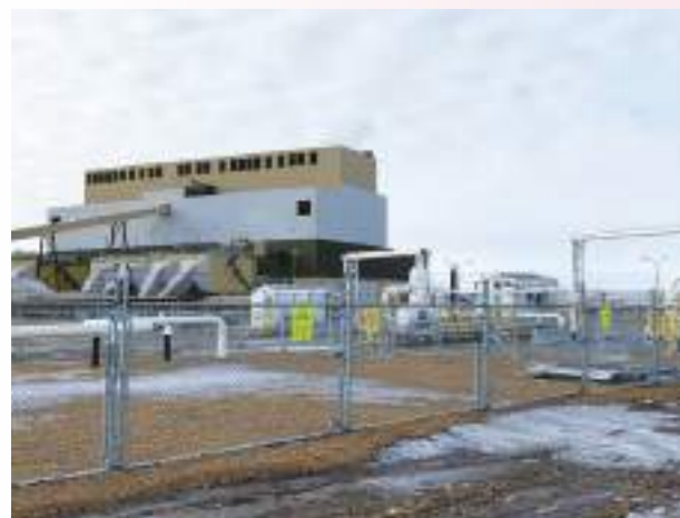
Sheerness Generating Station's gas receiving facilities
