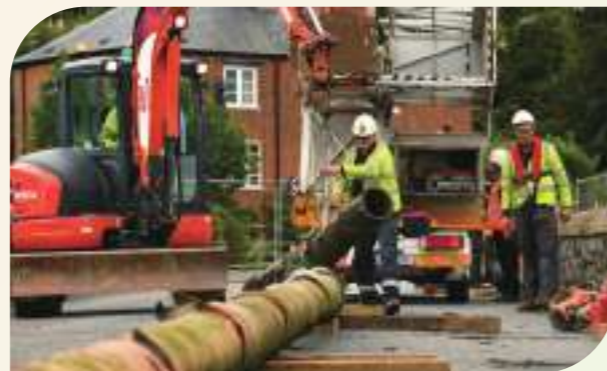
Workers replace legacy gas mains to eliminate emissions from gas leaks.
