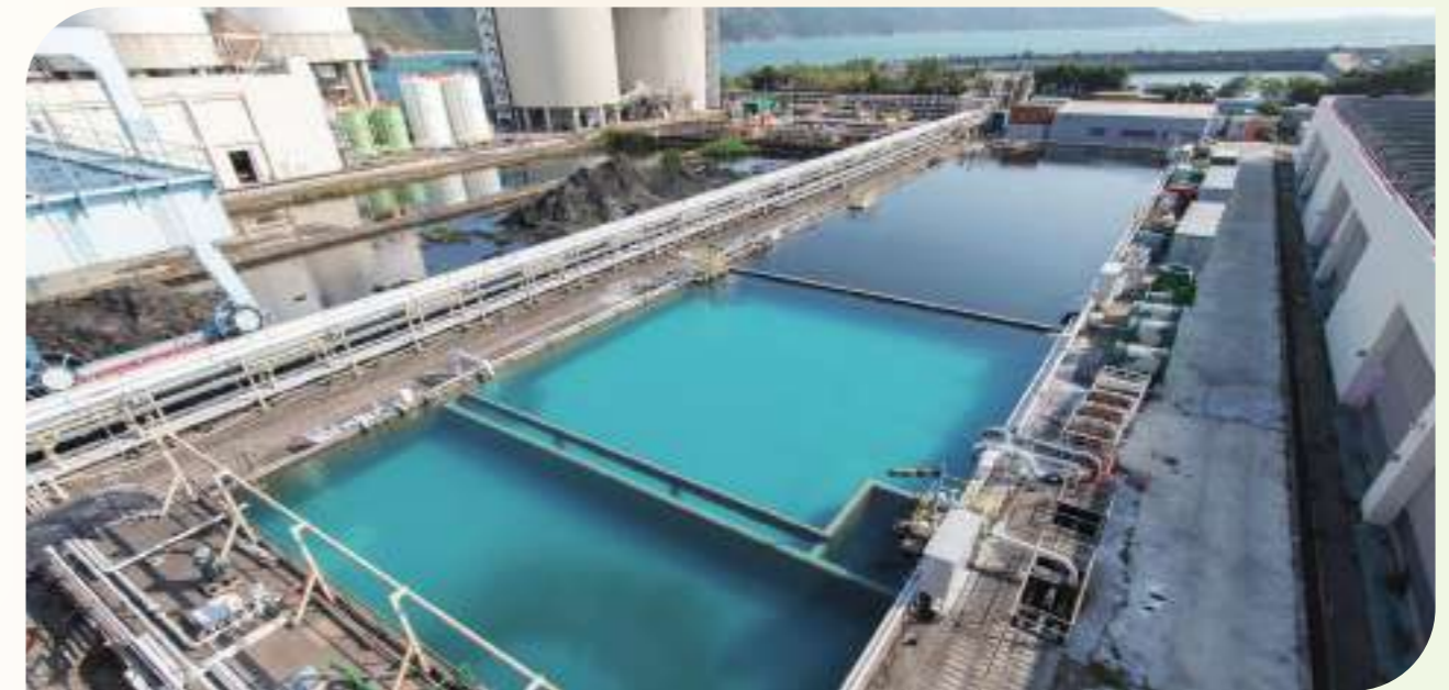
Rainwater and plant effluent is collected and reused at Lamma Power Station.
