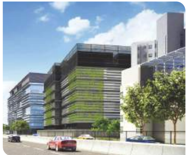
Artist's impression of the new IT Operations Building, scheduled for completion in 2024.
