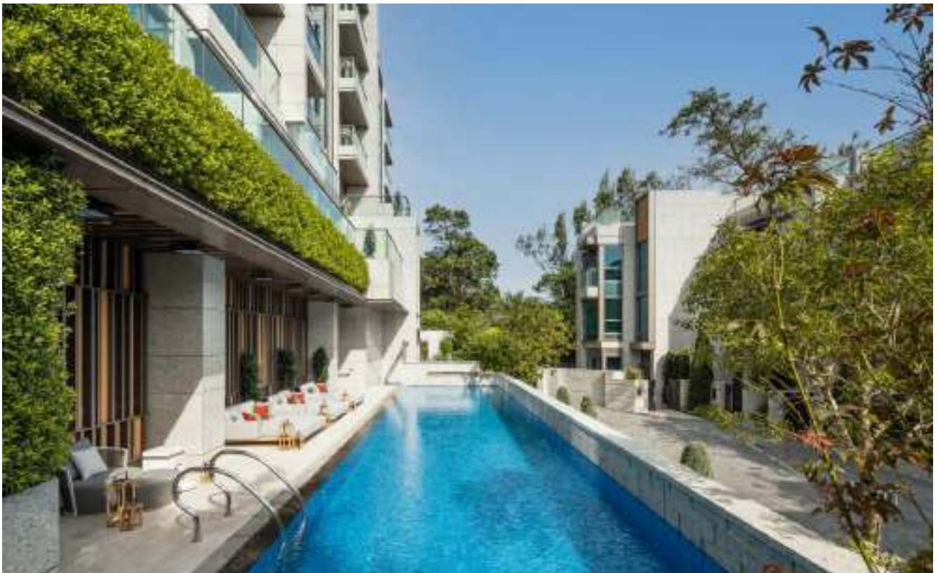
133 Portofino is one of our eight projects that has obtained WELL™ Precertification while under development.
