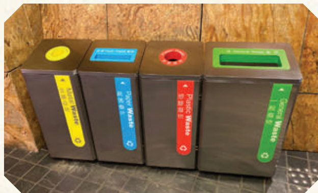
Sufficient recycling bins were installed at our properties to encourage recycling behaviours
