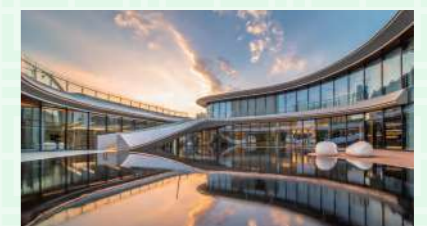
Hefei Shangdong District Project
