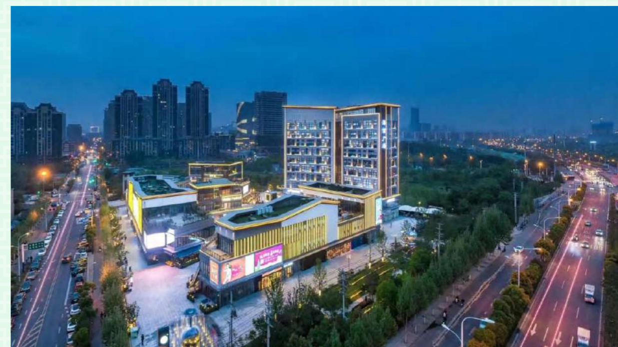
On-site Photo of Hefei Yangshu Huan Yu Tian Di Project
