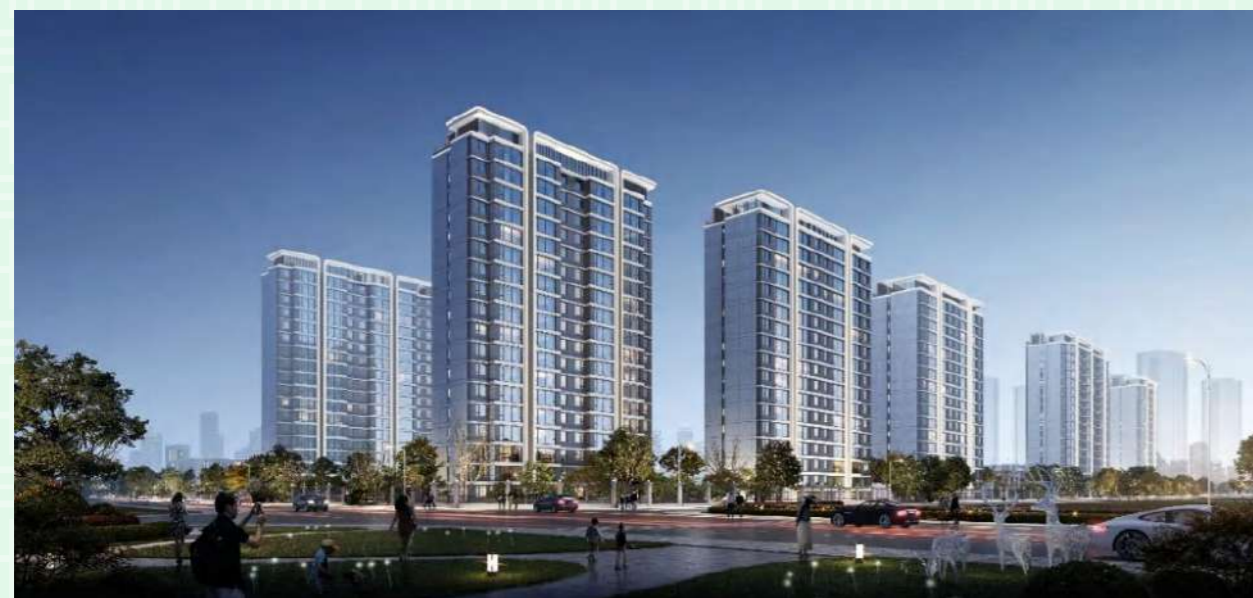
Xuzhou Huayue Project
