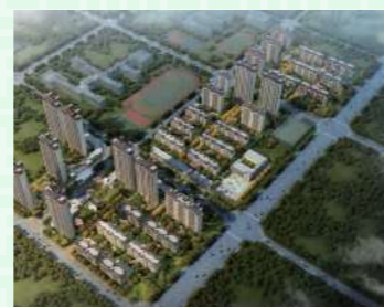
Jining COGO City Project
