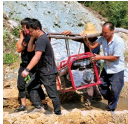
▲ Delivery of a diesel engine to a high-priority tower site
