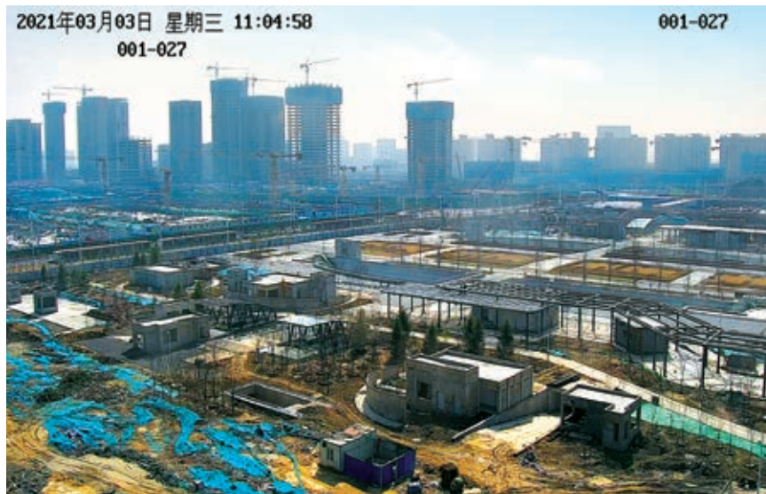
▲ The high-level intelligent video surveillance system
