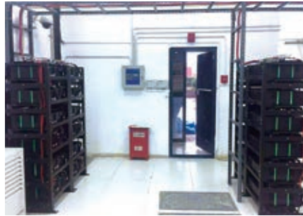
▲ Scenario of cascade utilization of power batteries for base stations
