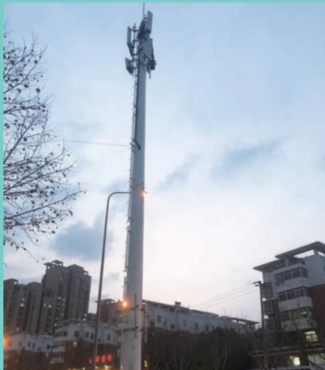
Site of height reduction and load increasing of low-load high tower
