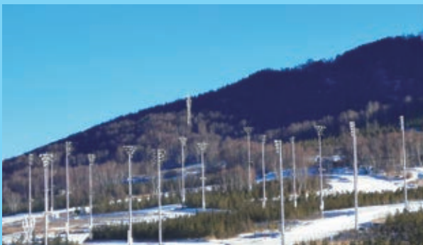
Construction of Tower Poles in the National Cross-country Skiing Center
