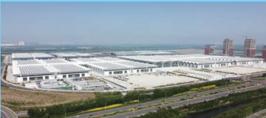
Full view of National Exhibition & Convention Center (Tianjin)
