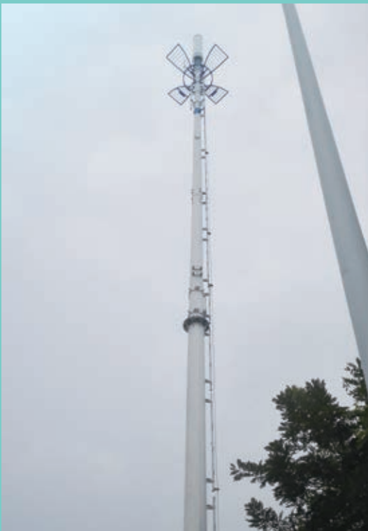
Site of height increasing of high-quality low tower
