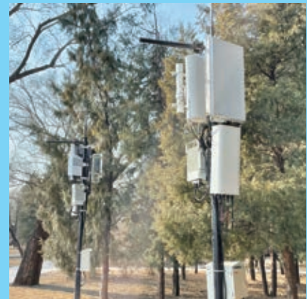
Achieving signal coverage in parks by using integrating local poles
