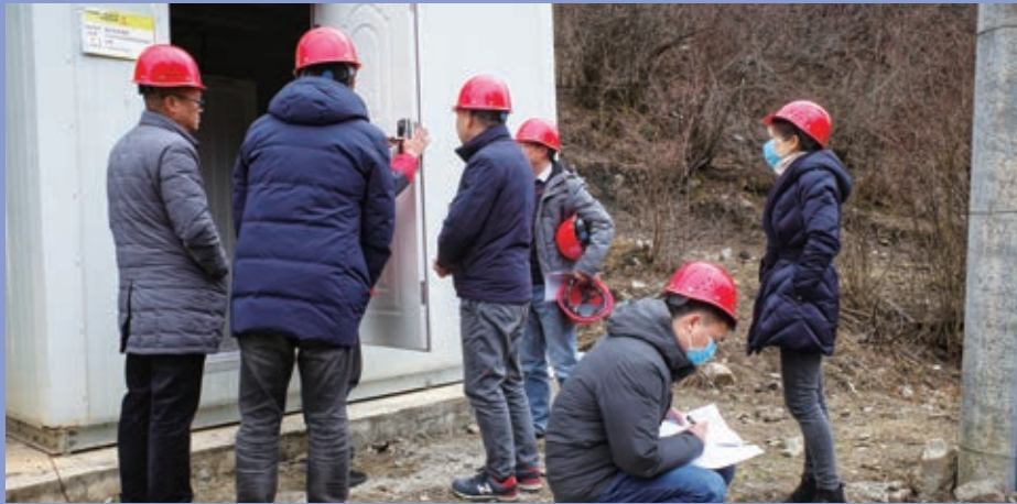
Rectification of existing towers
