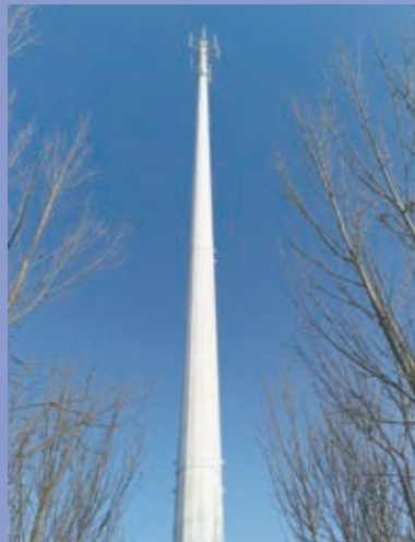
Example of low-cost single tube tower application
