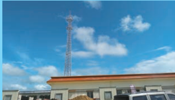
Deploying antennas on shared railway network towers
