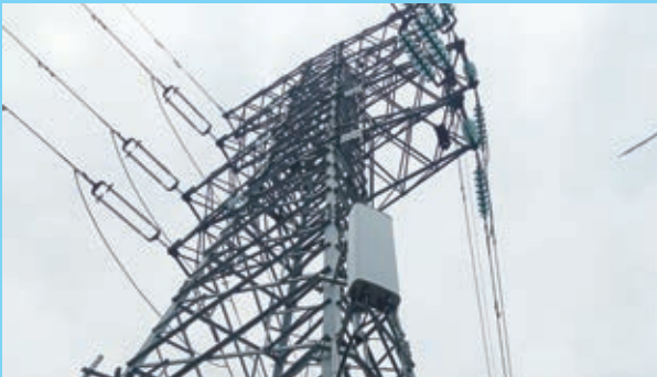
Mounting telecommunications antennas on 110 kV power tower
