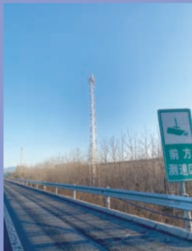
Example of low-cost three tube tower application
