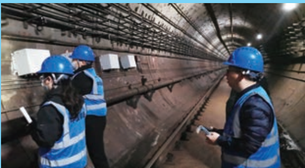
Construction of Nanjing Metro Network
