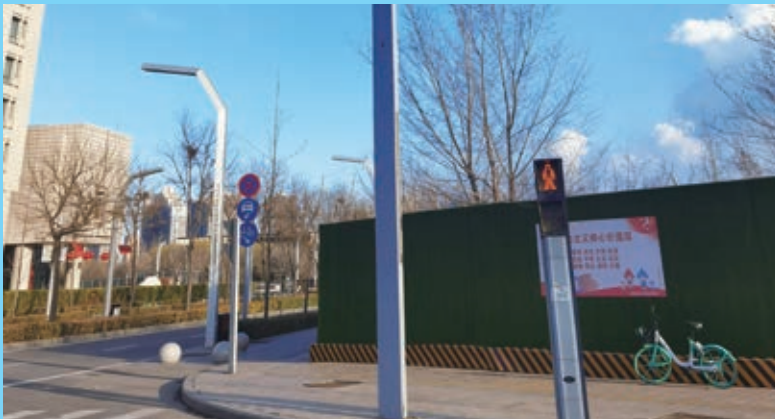
Improving 5G coverage in cities of Shanxi Province by using light poles
