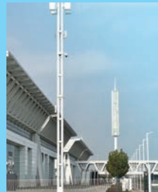
Construction of telecommunication towers using light poles
