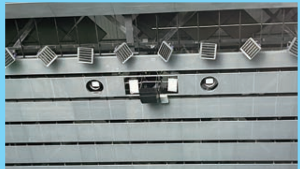
Internal Infrastructure in the Capital Gymnasium
