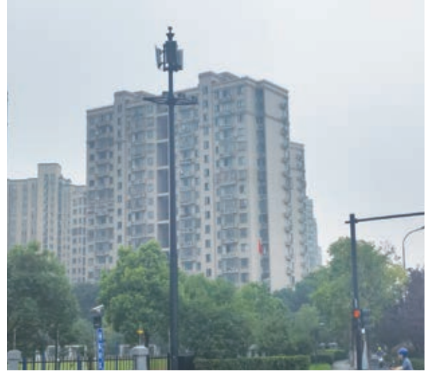
Replacement of mid pole lights
