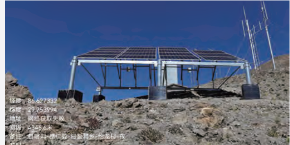
▲ Construction of solar base stations in Tibet
