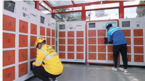
▲ The couriers use battery exchange service of China Tower
