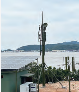
▲ The base station integrating solar energy, diesel, wind and storage in Putuo Mountain
