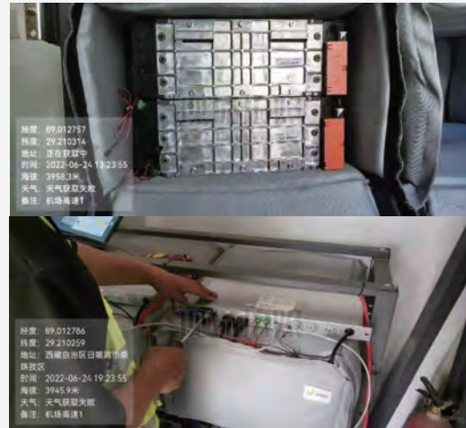
▲ Integrated intelligent communications & power backup cabinet
