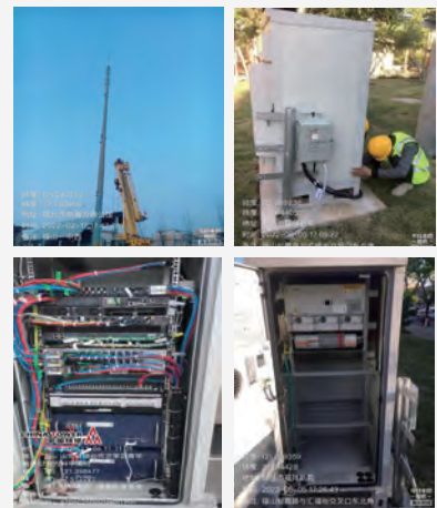
▲ Recycling site of dismantled materials
