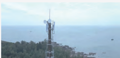
▲ Aerial view of the new materials tower
