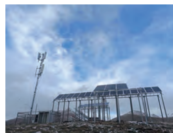
▲ Solar photovoltaic power supply for base station
