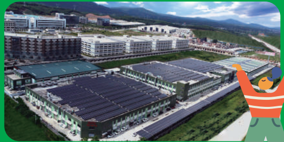
Installed solar panels at Kaiping factory
