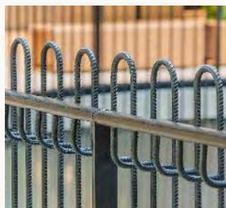
Railing made of recycled steel bars
