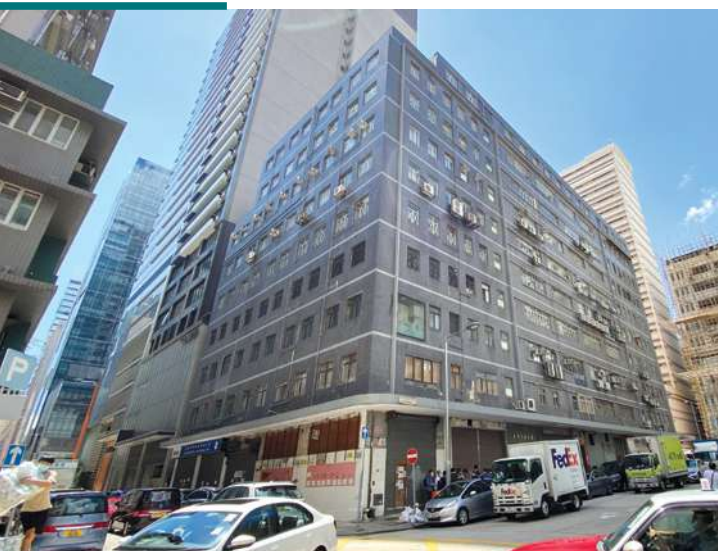
Retrofitting works to be carried out at Yu Chau West Street Project allows the URA to explore retrofitting initiatives to extend the serviceability of old industrial buildings.
