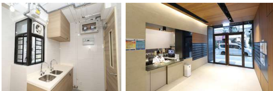
The flat units and facilities of the rehousing block at Soy Street are renovated to provide the tenants a more comfortable living environment.
