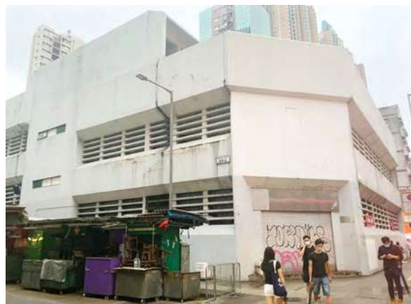
The ex-Mong Kok Market Building will be retrofitted into an interim District Health Centre for completion in early 2025.
