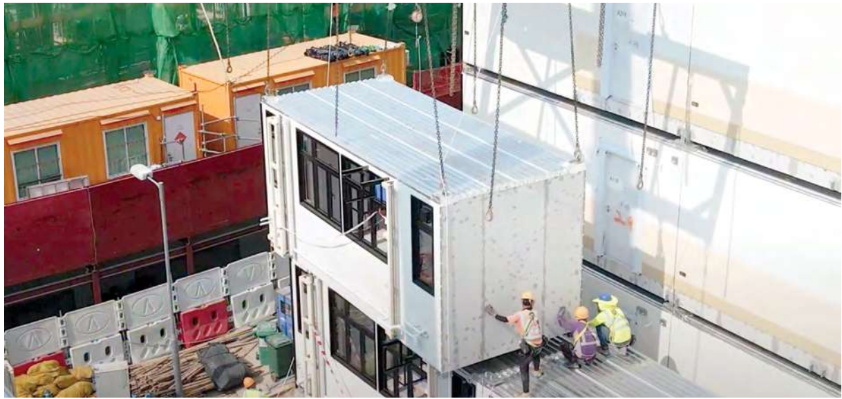
URA adopts Modular Integrated Construction (MiC) for the transitional housing project at Hung Shui Kiu for its sustainability benefits.
